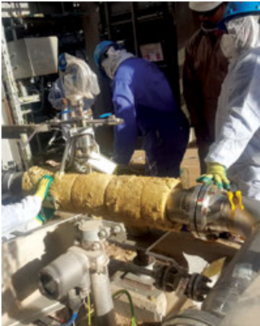
Painting and Insulation work for KOC LFHOD Project: EPC contractor Petrofac/Sinopec
